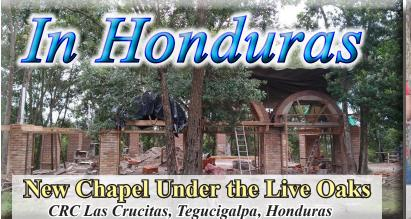
After months of building up the site with retaining walls, and tons of fill, and after hand pouring all the footings, we are finally seeing the 14 brick columns slowly rising up from the ground for what will be approximately a 45 x 68 foot open air chapel. The arches that connect the tops of the columns and will hold up the roof will be topped on two sides with large concrete and brick water channels.
